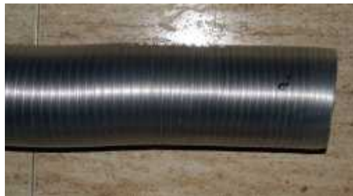
Straight with no bend is the most efficient
