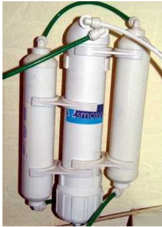
This reverse osmosis machine transforms water with a high ppm or EC into water with less than 10 ppm.
