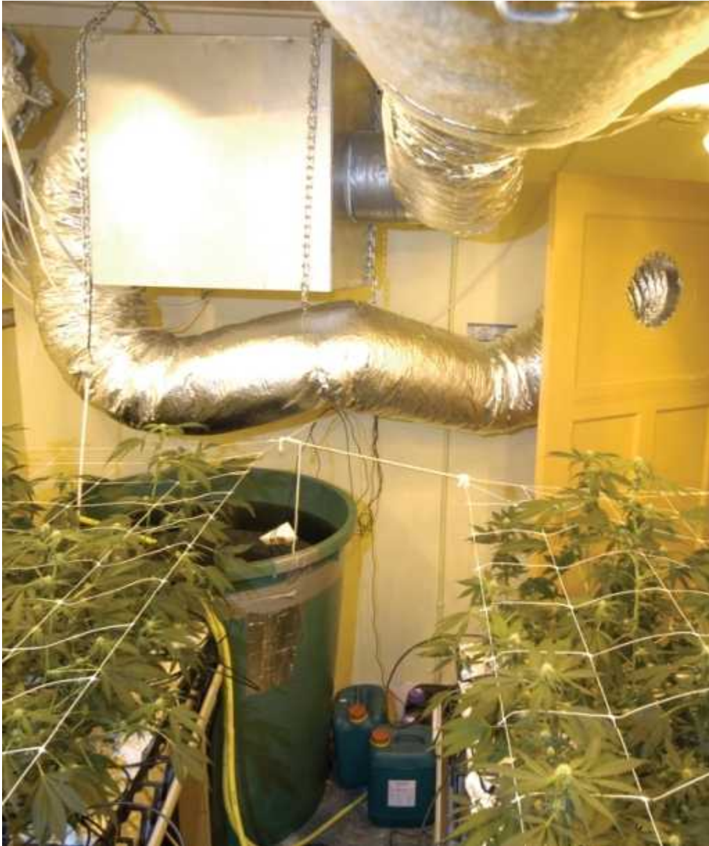
A carbon filter and ozone exchange box dominate the landscape in this Dutch grow room.
